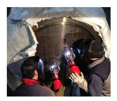
In tube to tube sheet applications, preparation is a very important aspect to guarantee repeatable and quality welding results. The following steps are discussed at each project and are essential to ensure the success of your process:
